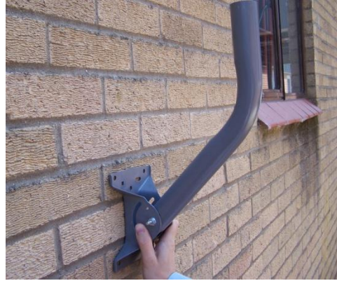
Figure 4-3 – Pole Assembly
